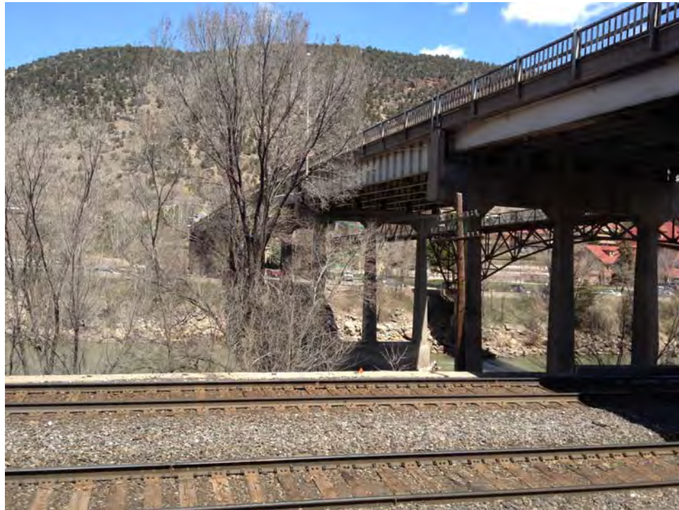
1. View to the North of the Existing Grand Avenue Bridge and the Colorado River.
