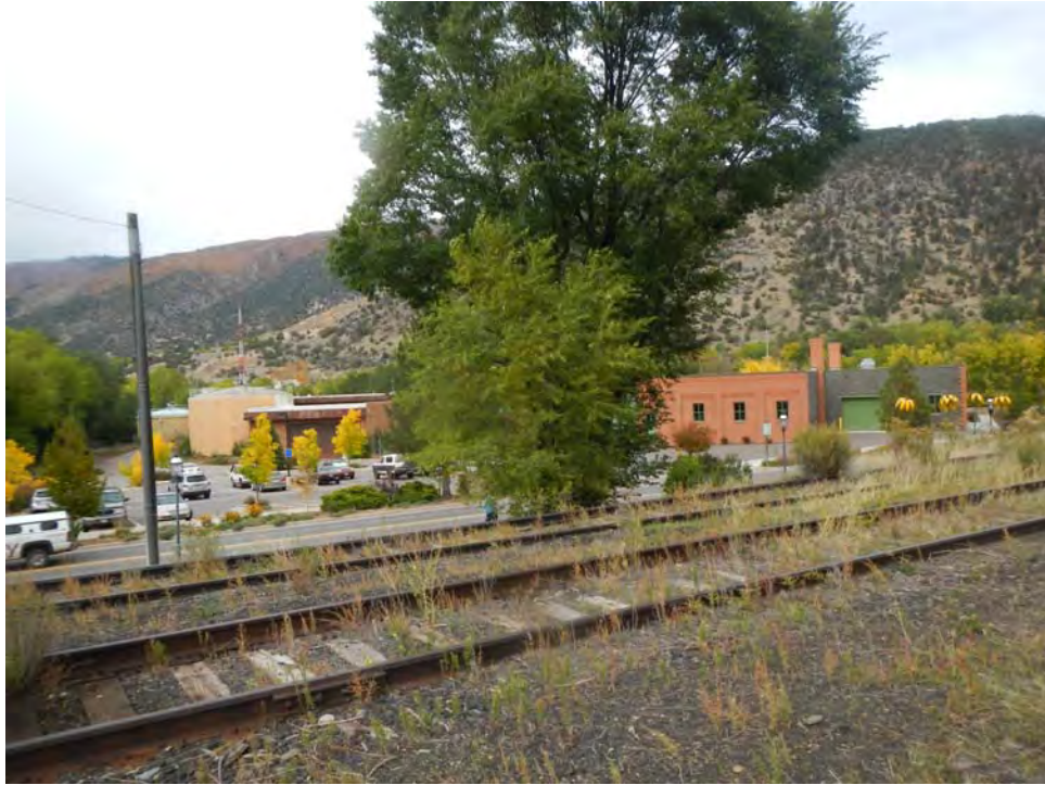
13. View of West 7 th Street and the Glenwood Springs Wastewater Treatment Plant, Facing Northwest.
